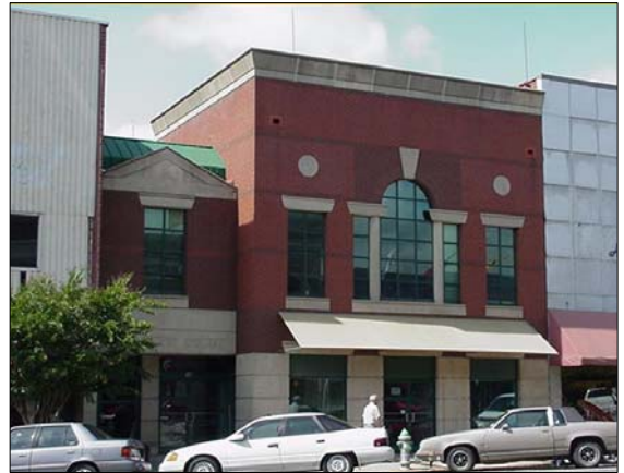
Contemporary new construction
