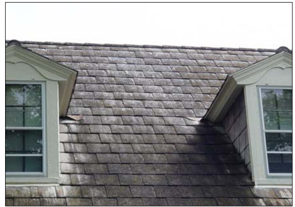
Replacement materials should match original in composition, profile, pattern, and size.
