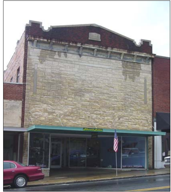
Removal of non-historic synthetic covering is encouraged.
