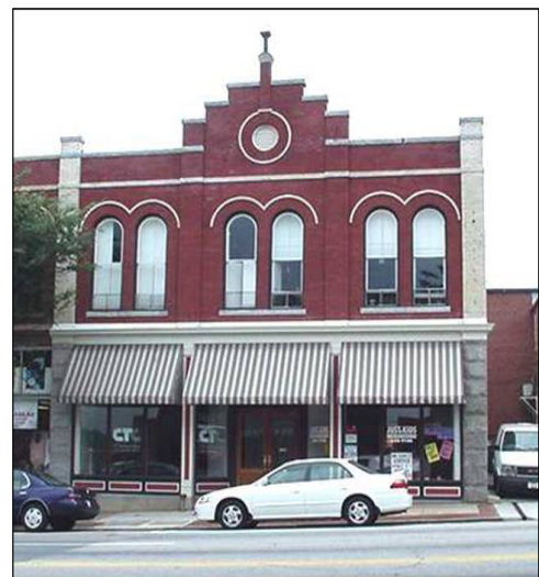
Reconstructed storefront based on original design
