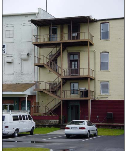
Fire escape and access accommodated on rear elevation.
