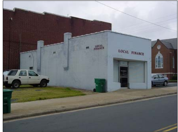
Commercial structures typically have flat sloping roofs.
