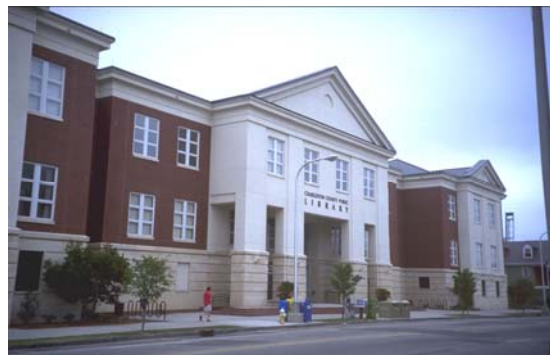
Compatible new construction
