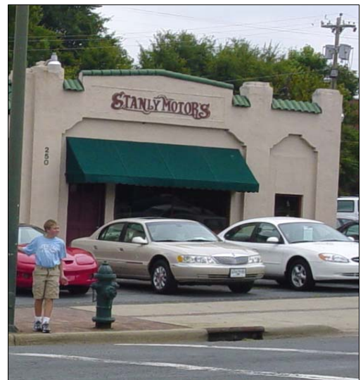
Stucco wall construction with terra cotta tile coping
