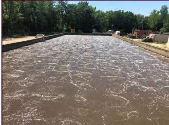
Fine bubble diffused aeration systems are designed to keep the wastewater completely mixed at all times, preventing dead spots from forming. All mechanical equipment is located away from the aeration basins in a blower building, providing for much easier, safer, and less expensive maintenance activities.
