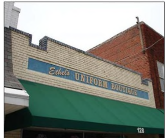
Wall signs should be flush mounted in appropriate locations above the storefront
