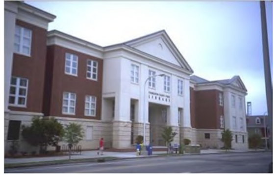
Compatible new construction
