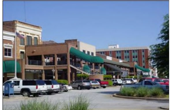
This addition to the front of historic commercial structures is incompatible in design and scale to the original buildings
