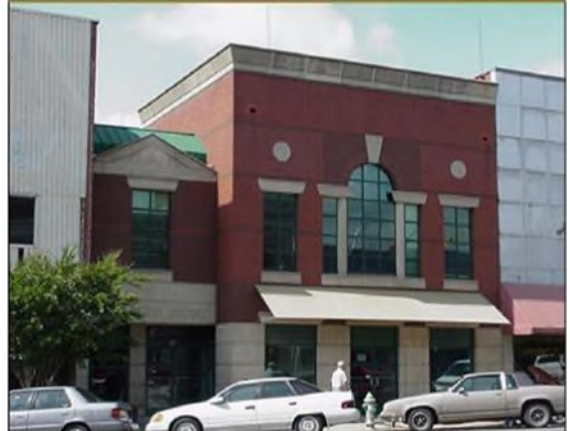
Contemporary new construction
