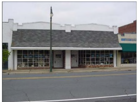
Continuous awnings, or awnings that obscure architectural features are inappropriate
