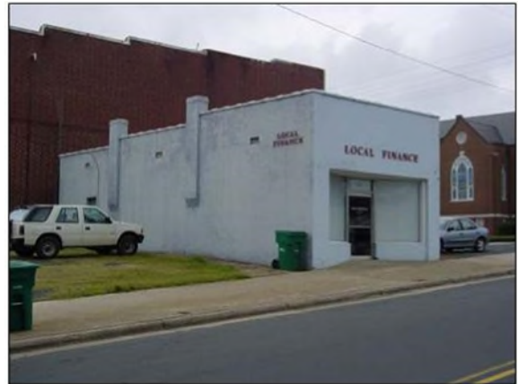
Commercial structures typically have flat sloping roofs.
