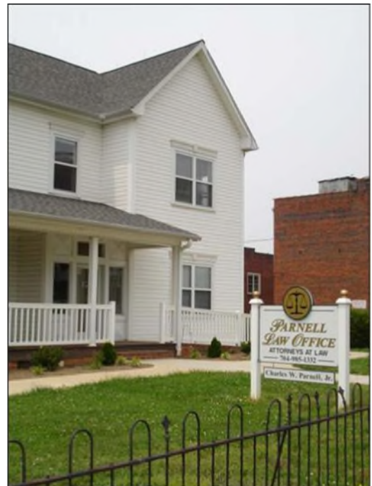
The size, style and location of signage should be compatible with the building’s architecture
