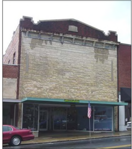
Removal of non-historic synthetic covering is encouraged.
