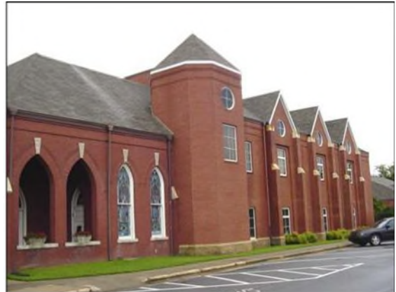
This addition to a historic church structure is contemporary yet compatible with the design of the main structure.
