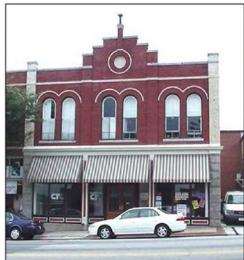
Reconstructed storefront based on original design
