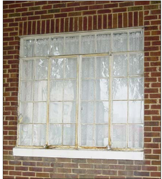
Preservation of original window units is encouraged
