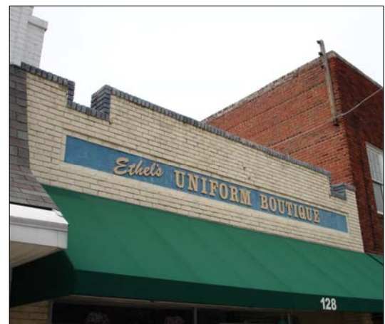
Wall signs should be flush mounted in appropriate locations above the storefront
