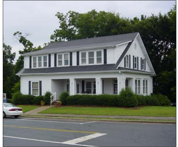
End gable with shed roof on front
