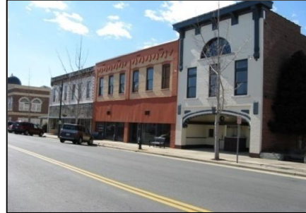
Downtown Albemarle Building Facades
